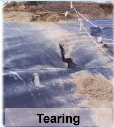
Damage during installation
