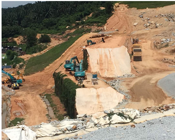
Free Standing Wall Flexible Geogrid Wall with two tiers
